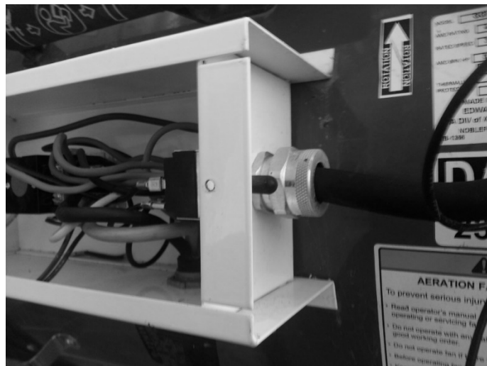
Figure 1: SOOW cable into aeration fan box
